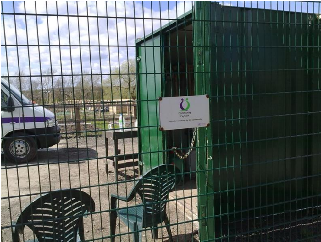
Figure 13: View of worksite from pavement
