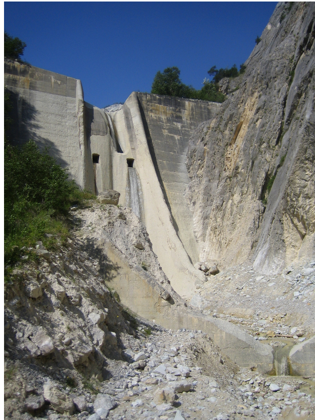
Figure A.4: The sediment retention dam (CD1) seen from downstream, total height is 40 m. Note abrasion of concrete structure by debris flows.
