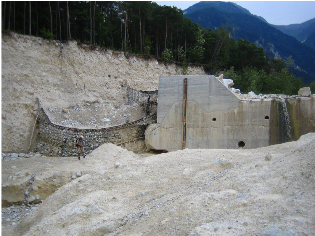
Figure A.12: Deeply incised active channel on the Illgraben fan. Stabilization and protection of damaged check dam due to lateral erosion and bank collapse with ring net barriers.
