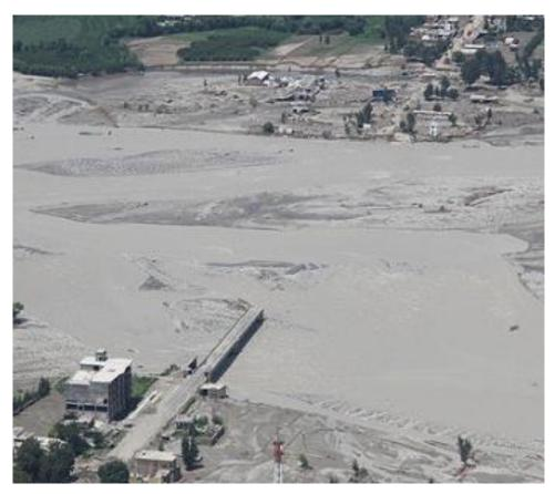
Figure 2.4: an example of a damaged bridge - Pakistan flood-2010 (adapted from EPACHA, 2010).
