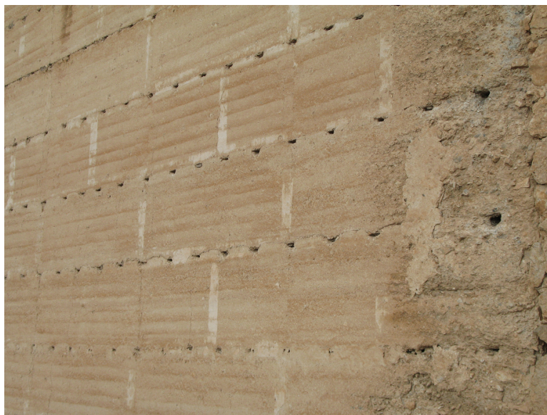
Figure 1.3: 12 th century RE wall (Castle of la Atalaya, Villena, Spain). Note the damaged material to the right of the photograph. Photograph by Paul A. Jaquin. Used with permission.
