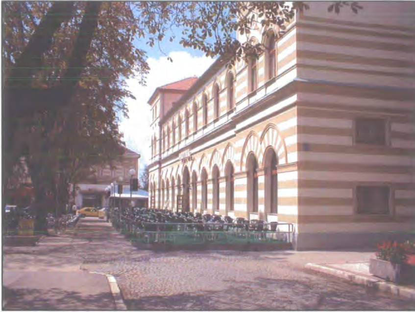
Figure 2.3 The Hotel Posavina, Brčko
