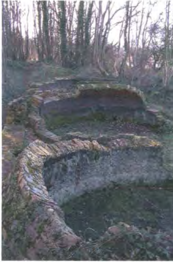
Fig. 91 Alongside coal, the Throckley Coal Company manufactured coke, mainly for use at Spencer's steelworks. A bank of twenty-two coke ovens was built using Stephenson's bricks, close to the Isabella Pit in 1869. They are shown on fig. 254. In 1875 the number of ovens was doubled and three years later a disintegrator for crushing the coal was added. In 1890 another twenty coke ovens were built. When new types of oven which could collect gases and by-products superseded the Beehive in the twentieth century, the complex went out of use (Ayris and Linsley 1994). These fragmentary remains of four beehive coke ovens survive in the woodland at Newburn Country Park (copyright author).
