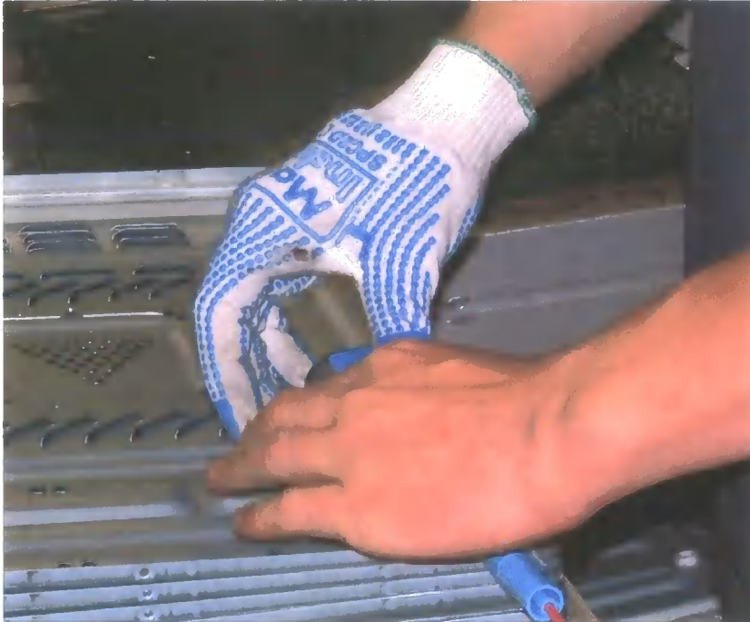
Illustration 5.4. The capacitor being clipped into place
