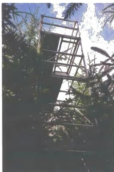
**Plate 7.1:** Photograph showing 6 m high scaffolding tower, with platforms at 2 m intervals.
