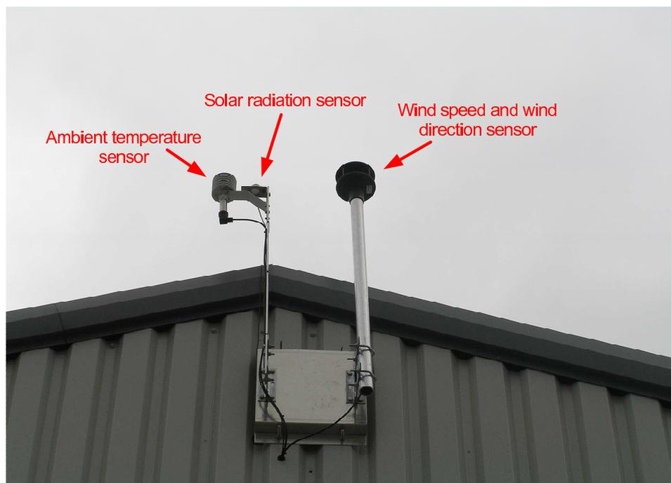
Figure 13.2: Meteorological sensors installed in the Rhyl substation compound
