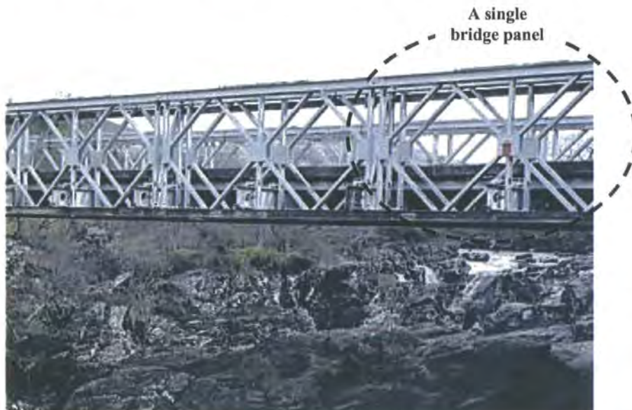
Figure 4.4: Bailey's Bridge – (Picture courtesy of Mabey & Johnson, UK)
