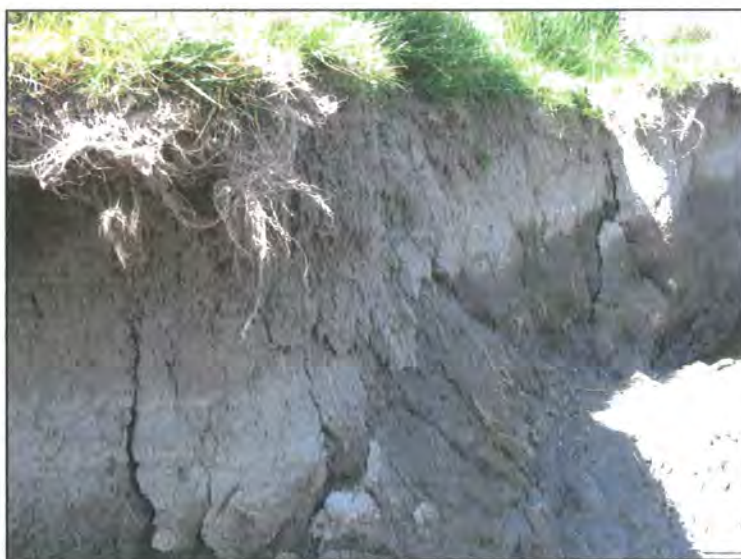
Figure 2.19: A desiccated river bank on the River Derwent near Bassenthwaite Lake, showing a dry and crumbly upper bank with deep cracks in the upper bank surface.
