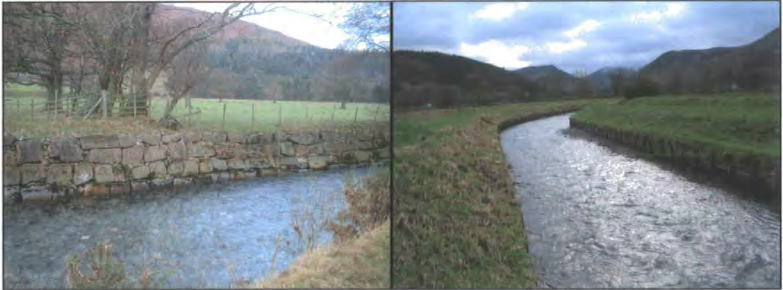
Figure 2.5: Channel regulation on Newlands Beck, showing channel straightening and bank heightening and reinforcement using (left) boulder revetments (NY 238 221) and (right) wooden revetments at Newlands Bridge (NY 240 263).
