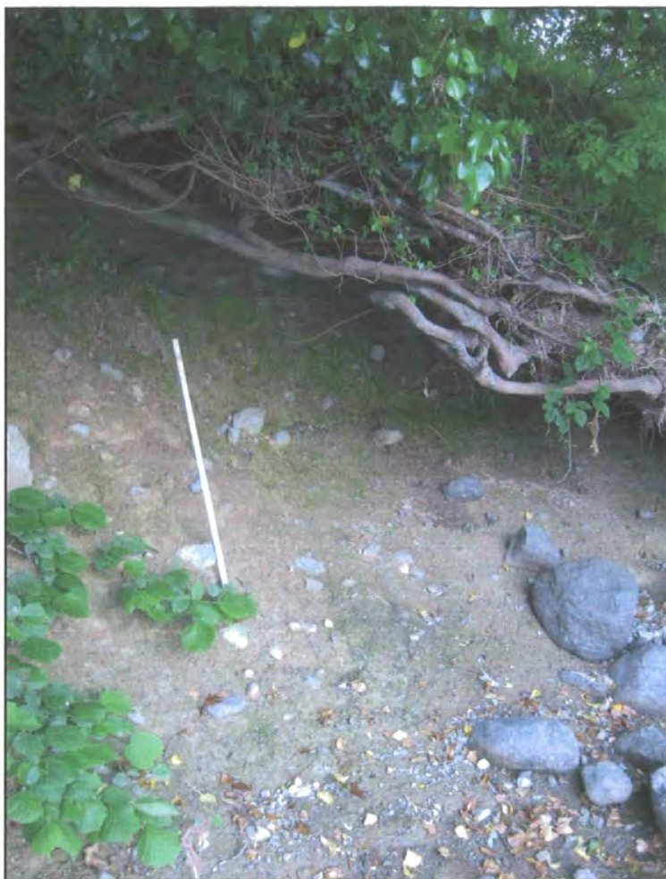
Figure 4.29: High (3.5 m) but presently stable river bank near Portinscale (NY 252 238), with metre ruler for scale. The dense vegetation roots at the overhang and the highly cohesive till on the lower, exposed bank face have prevented active erosion of this bank.
