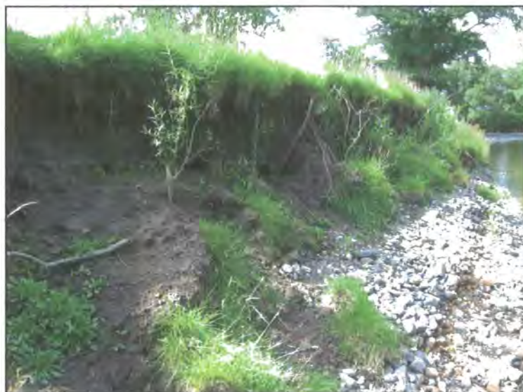
Figure 4.20: Bank 2 (West bank, NY 255 237, looking downstream).
