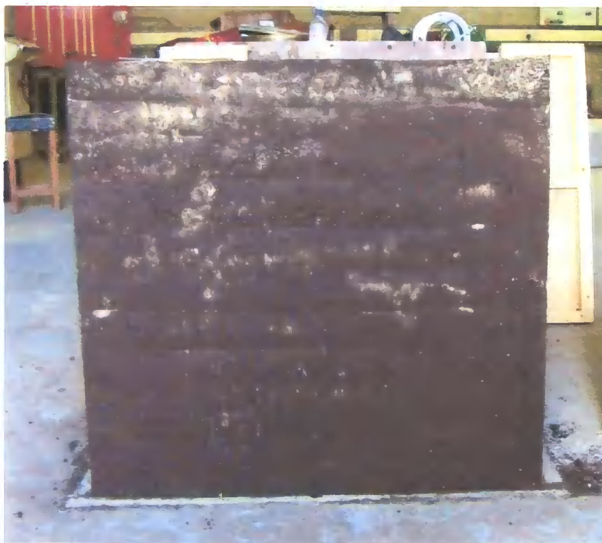
Figure 2.17 Wall 2 drying, 24/05/05, day 1
