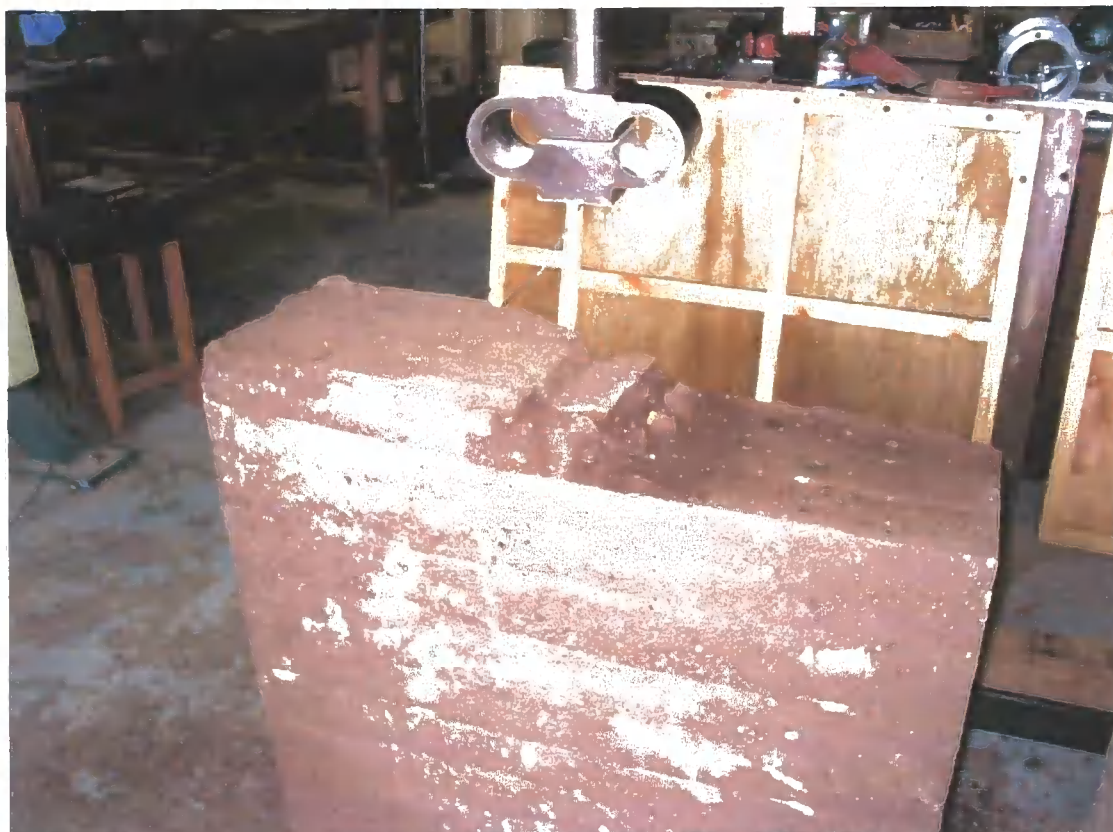
Figure 2.22 Wall 2.1 failure through delamination
