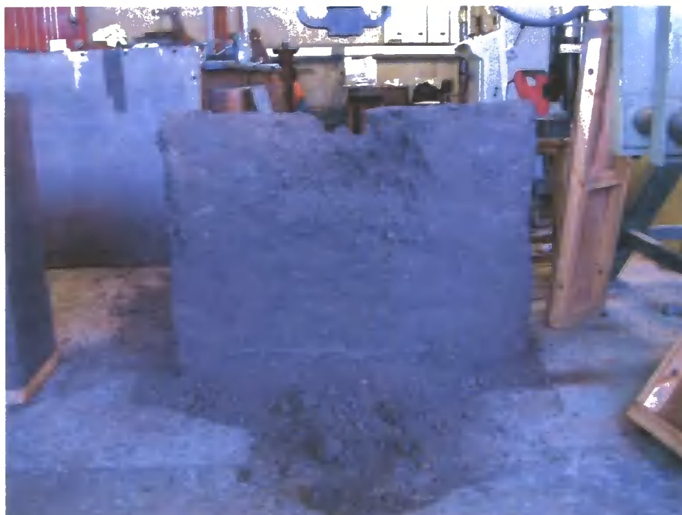
Figure 2.28 Wall 3 out-of-plane failure
