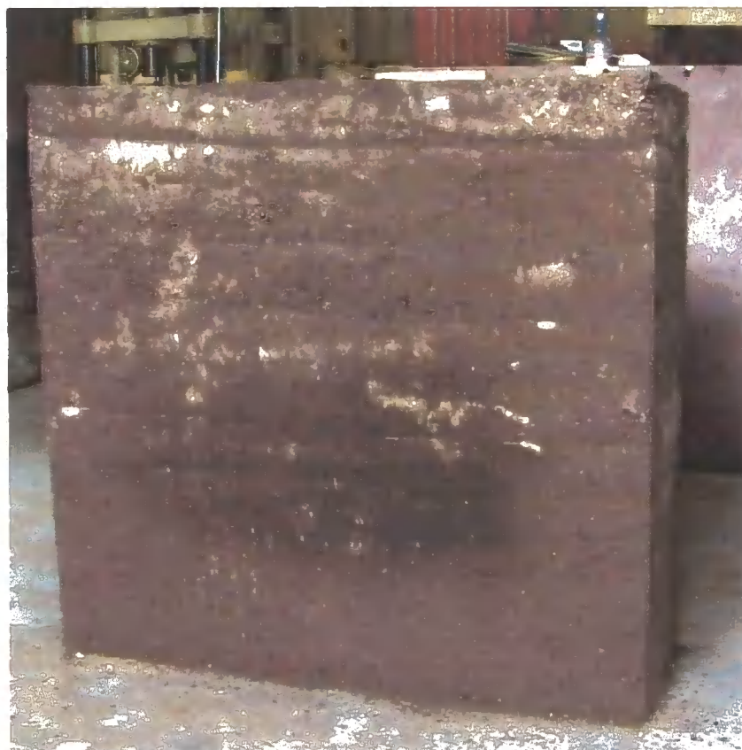
Figure 2.19 Wall 2 drying, 31/05/05, day 8
