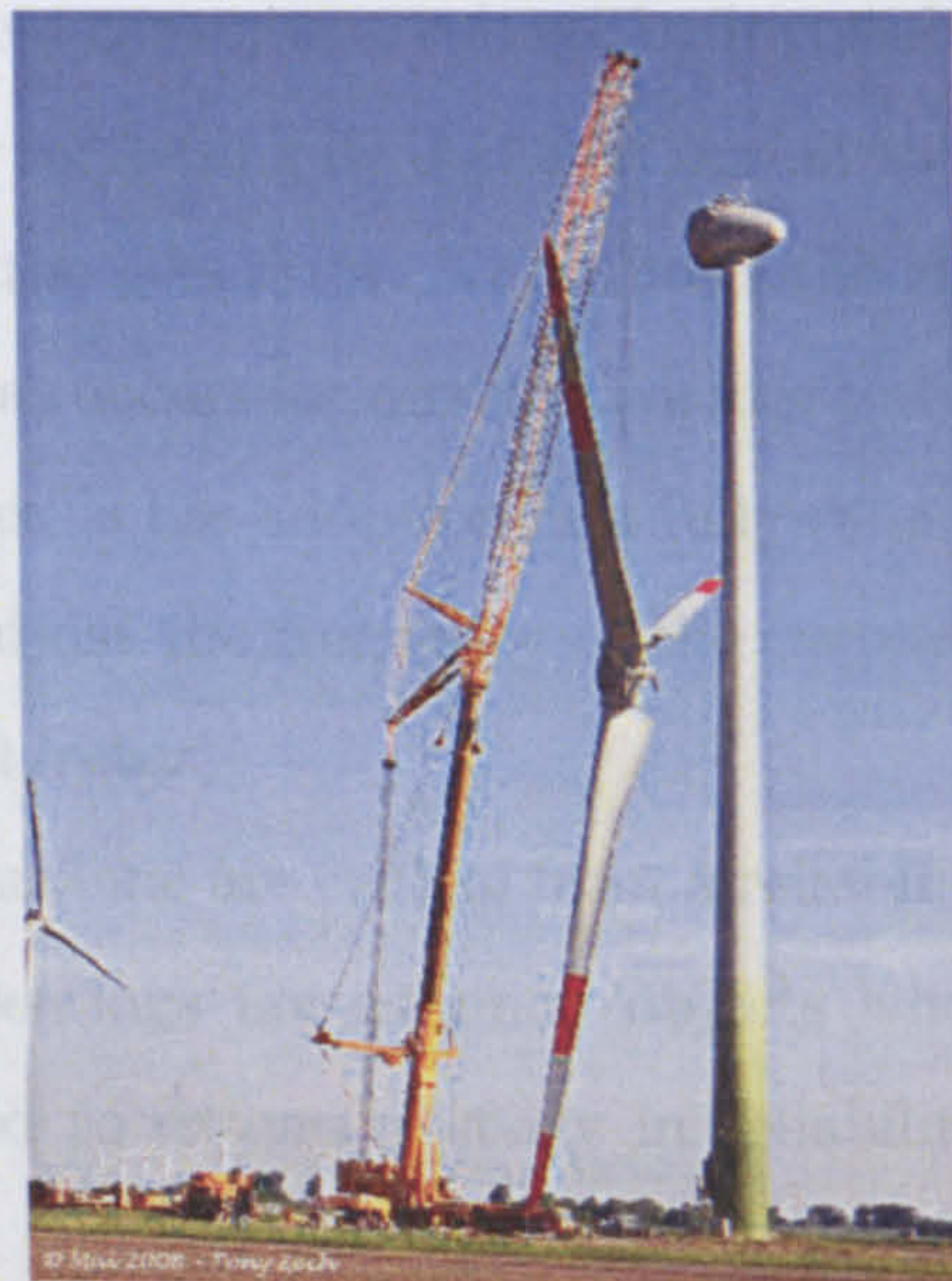
Figure 4.2: A rotor of a direct drive machine, being mounted on the nacelle [66]
