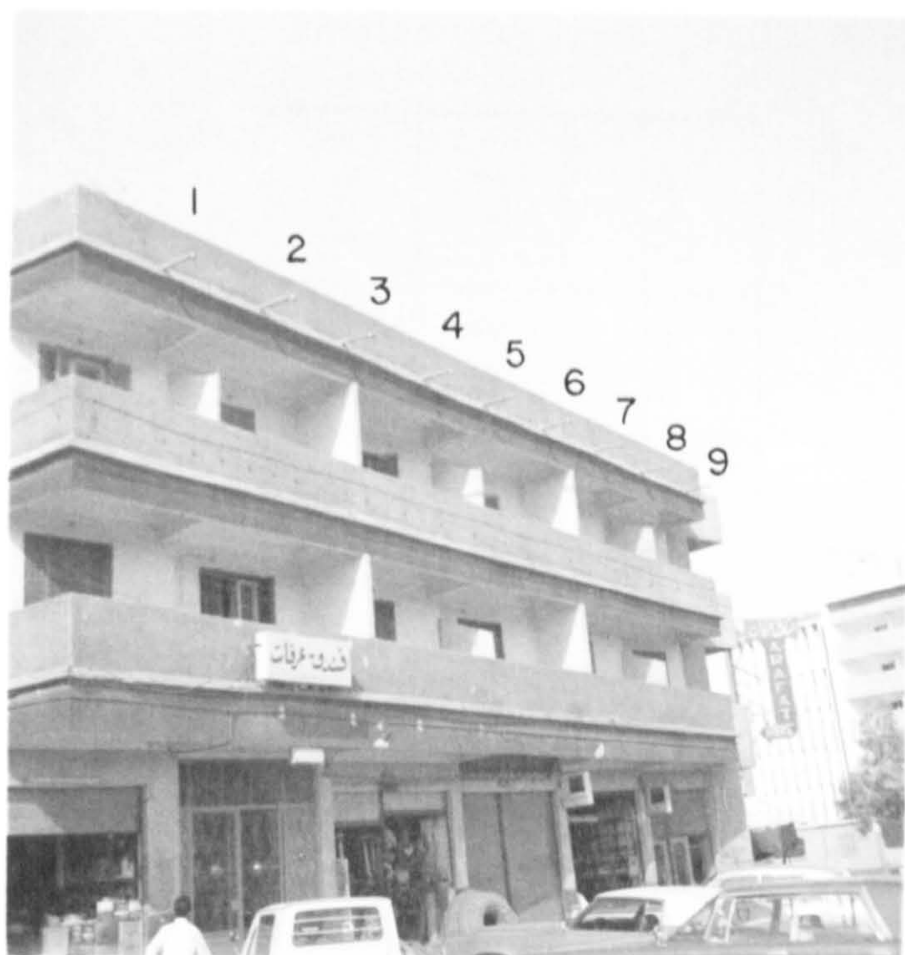
Plate 1.7 Roof equipped with several gutters. Arafat Hotel, At-Taif city Page 28
