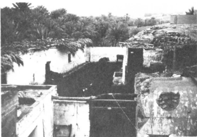
Plate 8-6 Areas provided for animals are small and sanitation is lacking (Deriyah, Riyadh).
