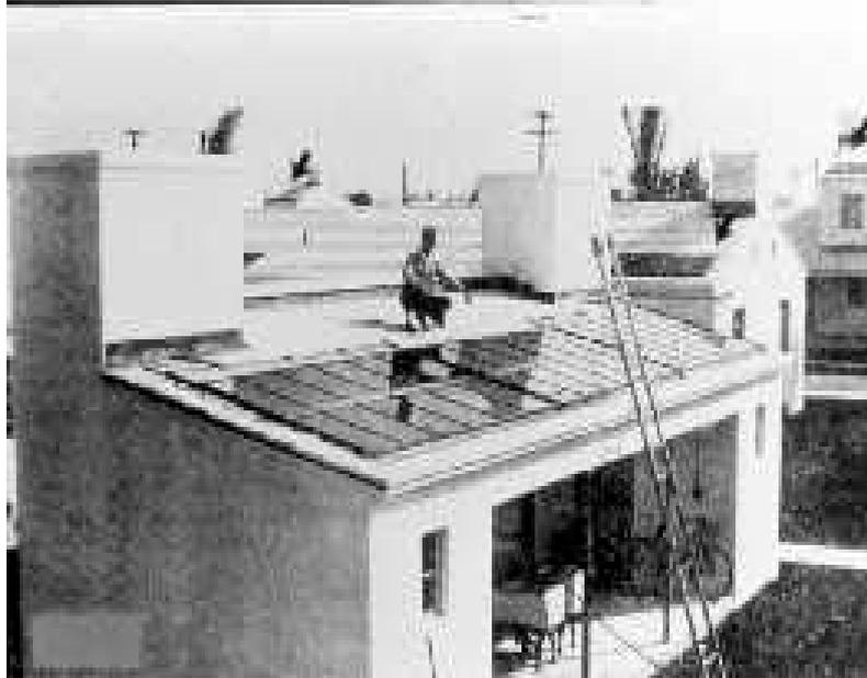
Figure 2.1b Solar water collector with separated storage tank [6].
