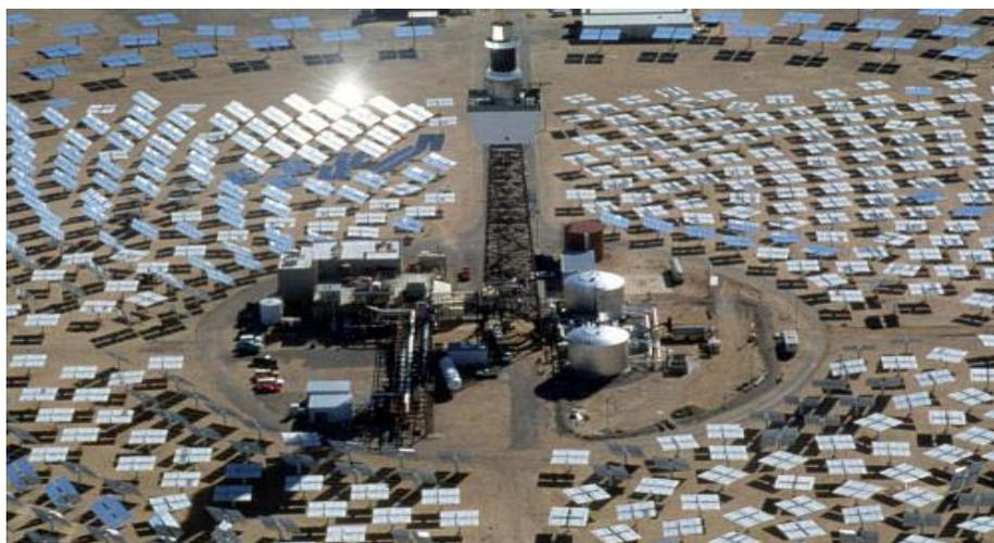
Figure 2.6a A Central Receiver System [13].
