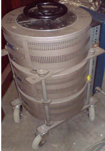
Figure 6.2d A three phase electrical transformer.
