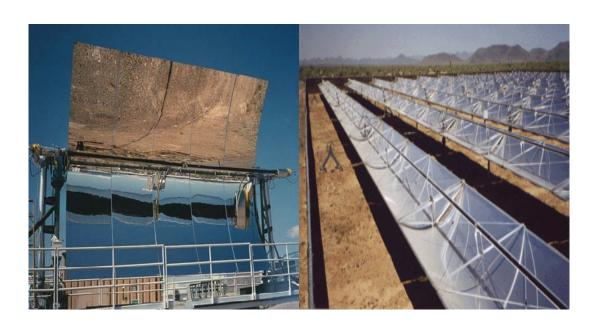
Figure 2.6c Parabolic trough collectors.
