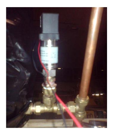
Figure 6.4e Pressure transducer.
