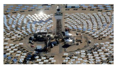
Figure 2.6a A Central Receiver System [13].
