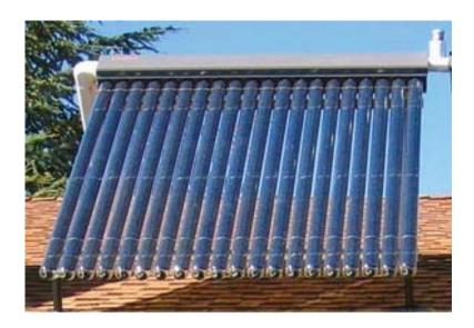
Figure 2.4a Evacuated tube collector.
