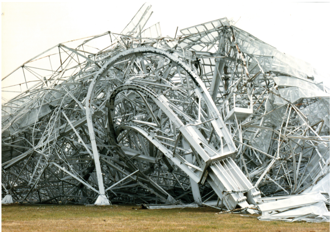
Figure 2.1: Photograph taken in 1988 of the collapsed 300-foot Green Bank Telescope in West Virginia. This incident highlights the engineering limitations of constructing large single dish telescopes to achieve higher angular resolution. Credit:NRAO/AUI/NSF.
