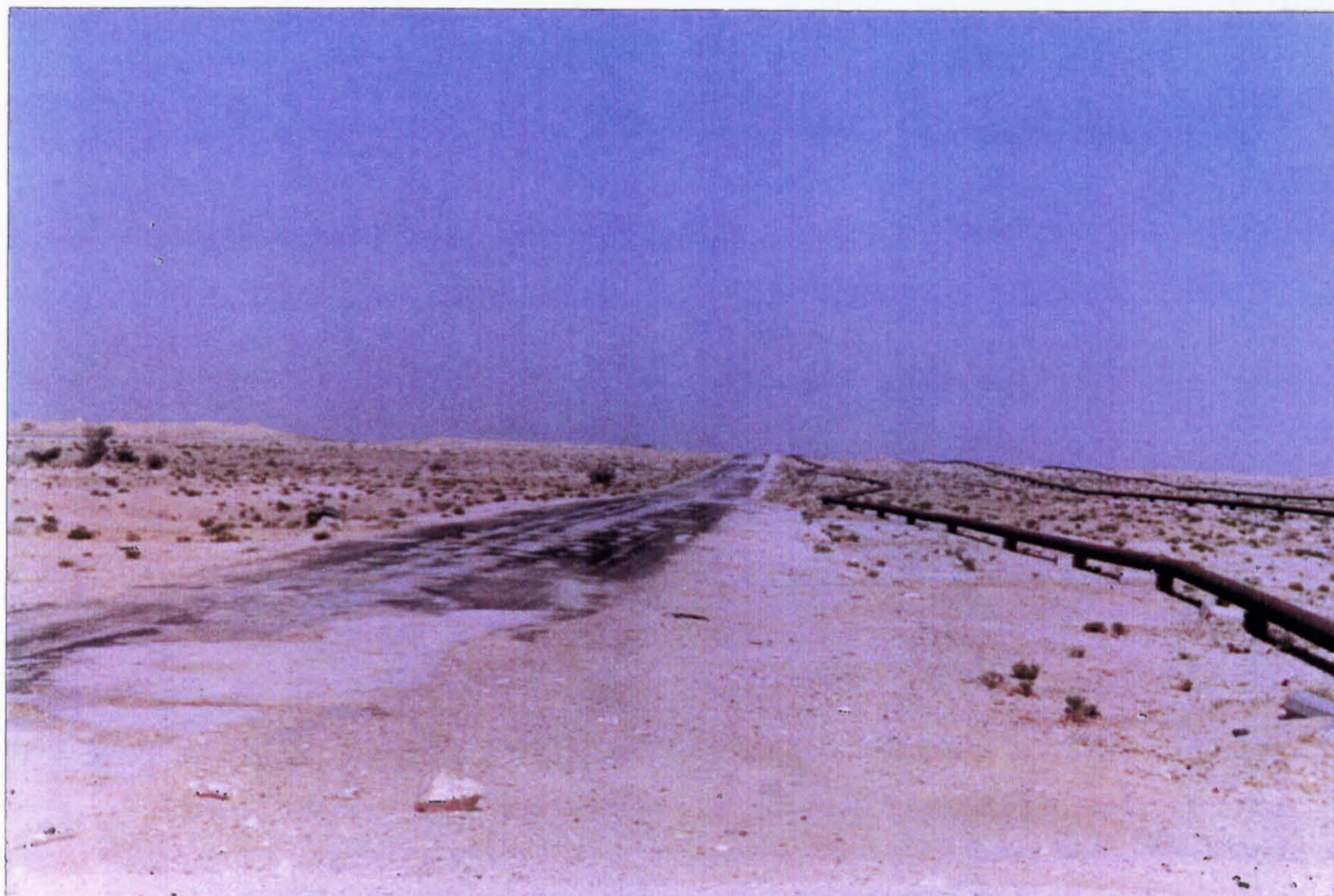
Plate 4.8: This road was built in 1947/48 for laying, maintenance and patrolling the first regional pipeline in Qatar's history, between Umm Bab and Umm Said.
