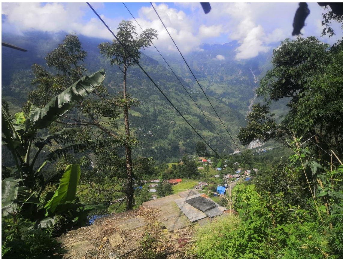
Figure 5.5: Drinking waterpipes elevated to prevent damage on pipelines from slumps and landslides
