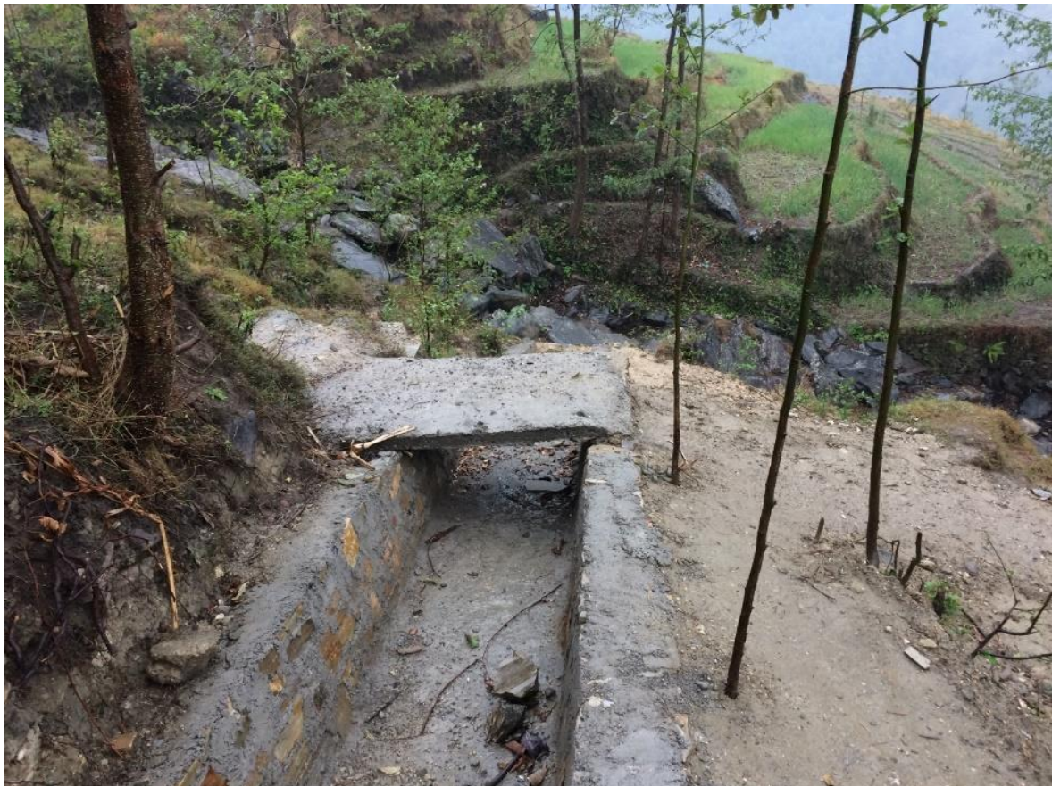
Figure 7.18: A drain cemented on base and sides to minimize infiltration and diverted towards natural rivulet in Tallo Sigarche
