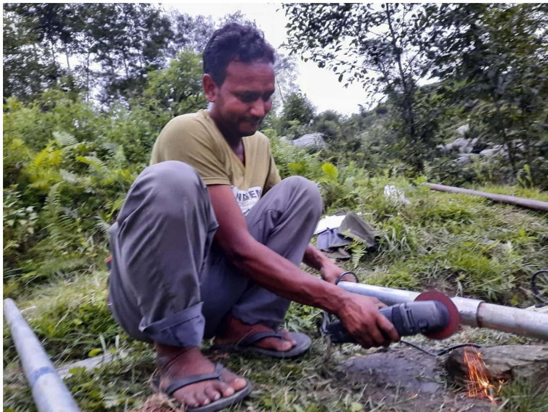
Figure 6.13: Birkha Shrestha, a local inhabitant of Tallo Sigarche, helping with smoothening the sockets connecting pieces of GI pipes to be used as wave guide for acoustic emission sensor
