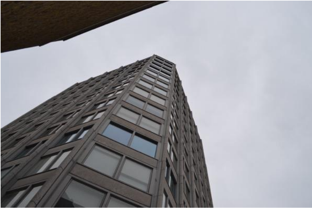
Fig.90 Smithson Building. Photograph by the author.
