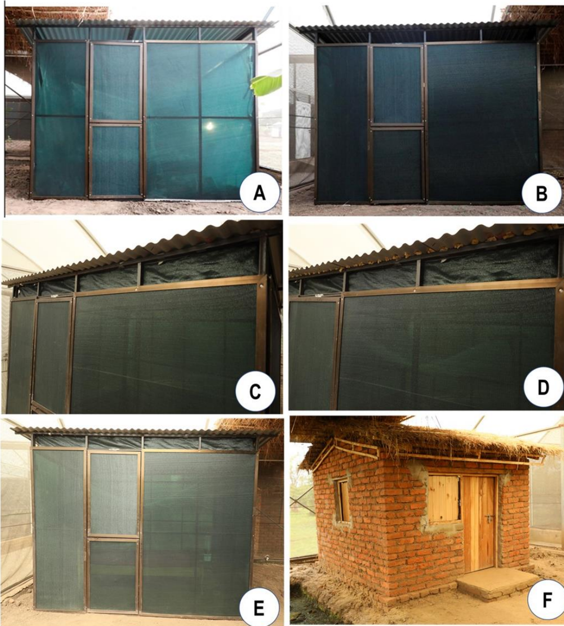
Appendix 1: Huts used in the study; opaque-walled, (A), transparent-walled houses, (B), partial open eave-gaps, (C), completely closed eave-gaps, (D), Star home-style house (E), and traditional-style house (F).
