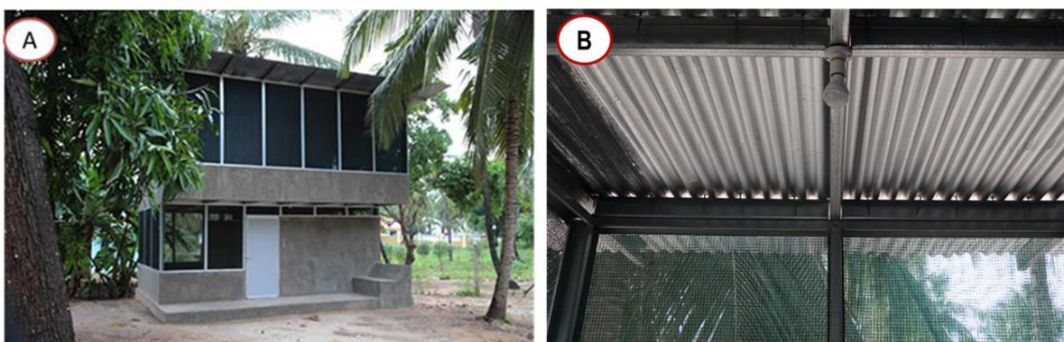
Figure 2.1: Star home. A, exterior view; B, interior view showing the air-permeable green shade-net wall and the bright light above the purlins and below the corrugate iron roof showing the openings under the roof.
