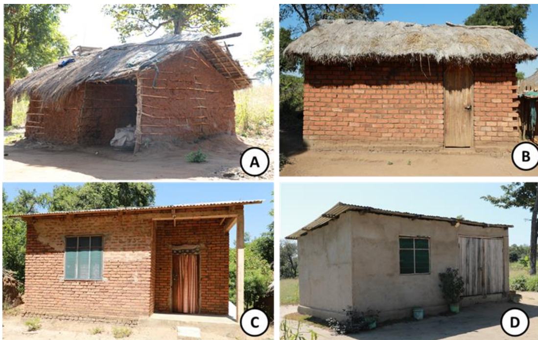
Figure 1.1: Transition of housing improvements in rural Tanzania villages; mud-walled with thatched roof, A), brick-walled with thatched roof, B), un-plastered brick-walled with corrugated iron roof, C) and plastered with corrugated iron-roof, D.
