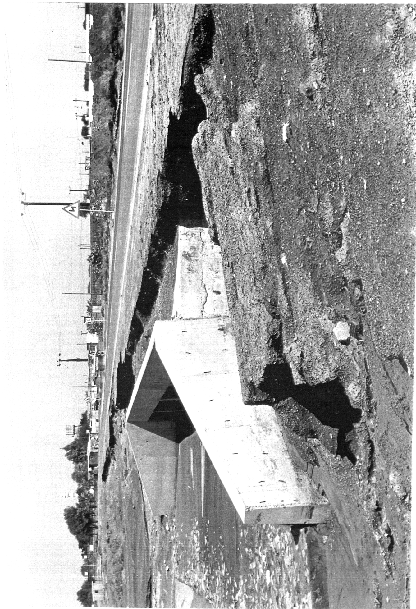
Fig. 3.4 Rain erosion on the slopes of embankments on the road of Manama - Ras al Khaimah.
