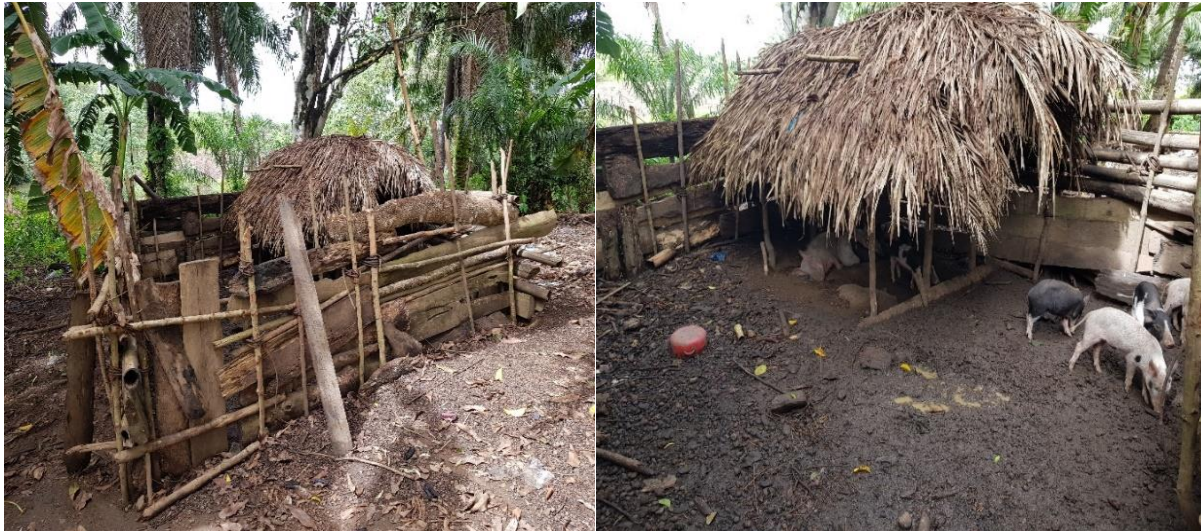
Figure 19. A pig pen built with tree branches, bamboo and timber waste.
