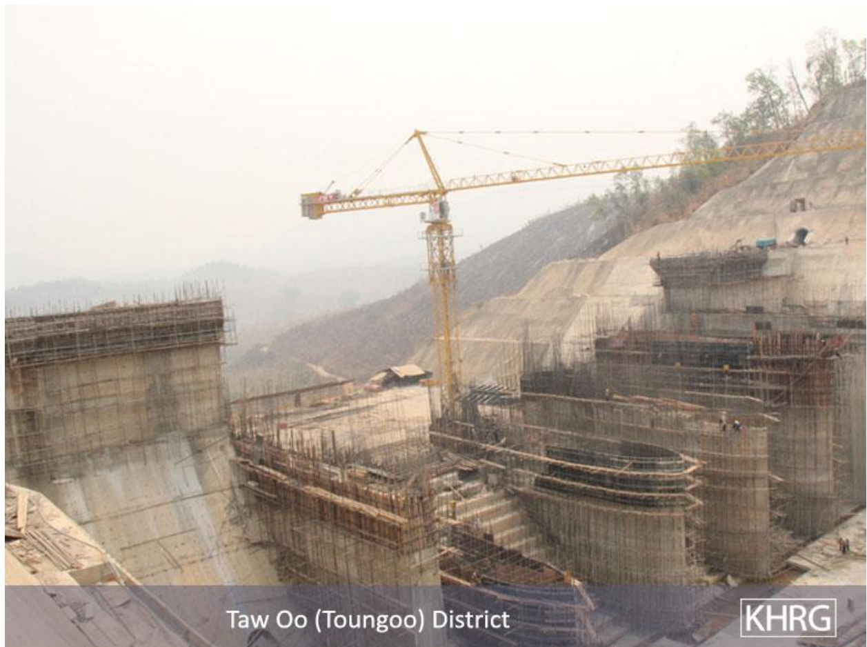
Photograph 1: Construction of the Toh Boh Dam (Karen Human Rights Group, 2012).
