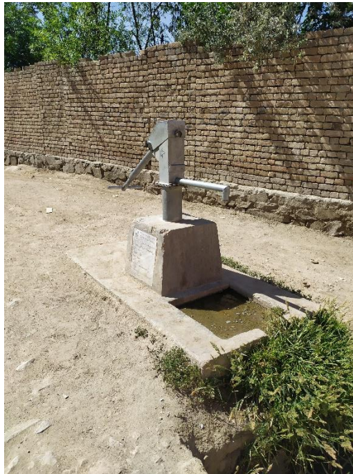
Figure 5.3 A handpump in the Bagrami area, built by NGOs, was not used due to the high salinity of the water.
