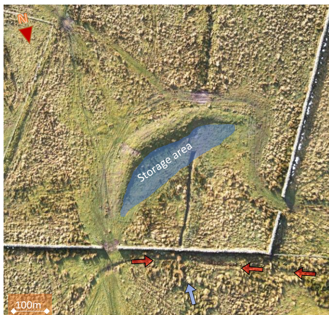
Figure 6. Aerial view of bund M14 (see Fig.4 for location). As shown, a secondary drainage ditch (indicated by the red arrows) runs parallel to the wall collecting further runoff from the field and discharging it into the main ditch (marked by the blue arrow).
