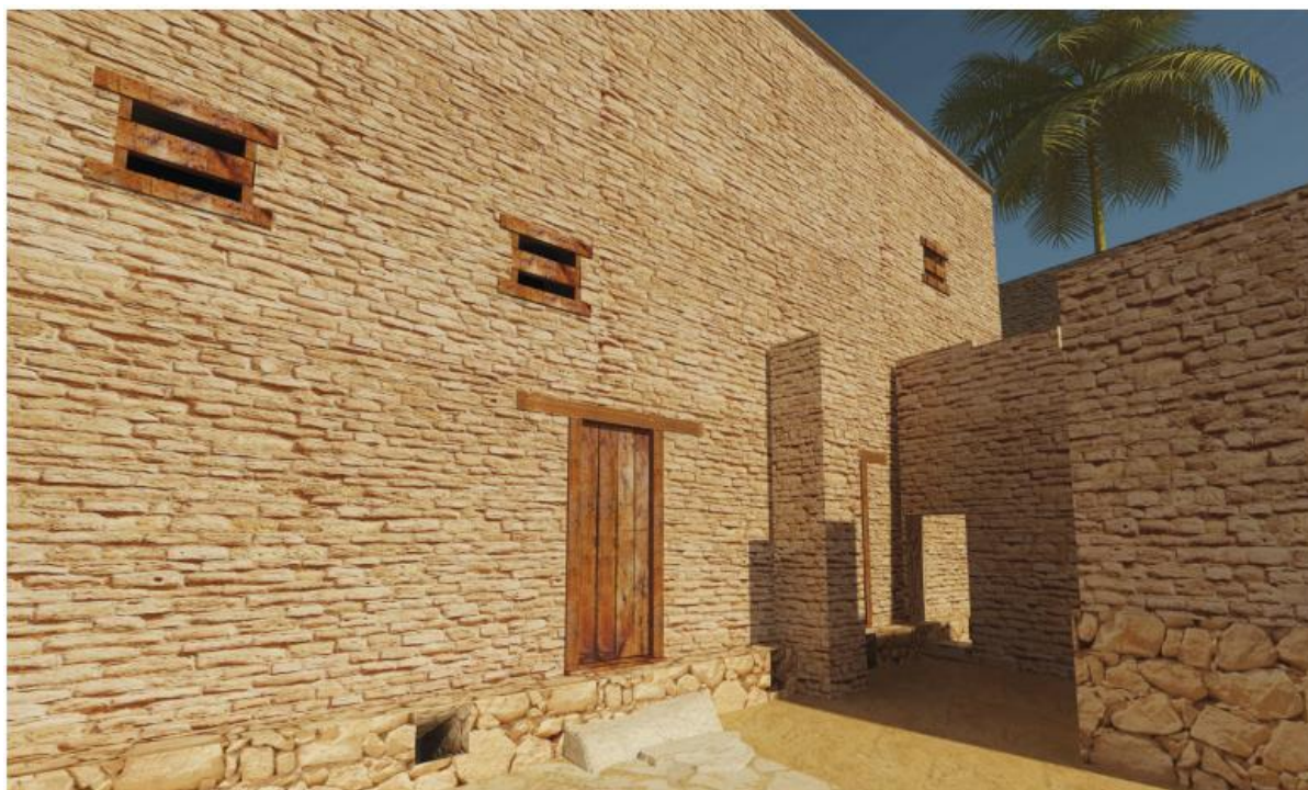
Figure 140 The 3D reconstruction of Karanis House C45 was depicted with straight rather than concave brick courses (Wendrich, Simpson and Elgewely 2014: 236, figure 5). Presumably, this is how a house would have looked like just after construction.
