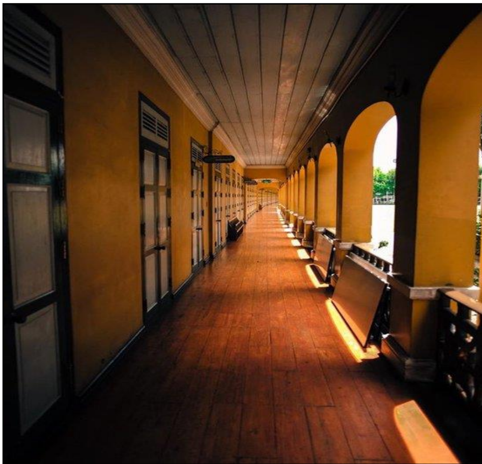
Figure 6: Ground floor colonnade of the Long Building as seen from reception room
