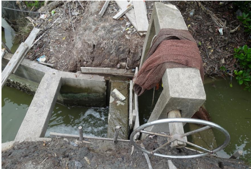
Figure 40 A sluice gate between the shrimp pond and the river
