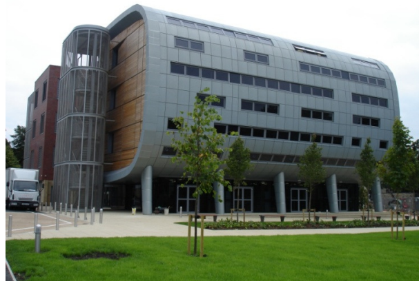
Figure 1.2 - Leeds University 2005, showing the impact of aesthetics using curved metal sheet cladding on a building design, this project was manufactured by PSP Architectural Ltd., see Appendix A.
