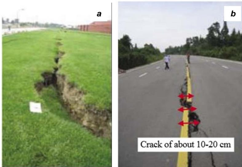
**Fig. 2.08:** Examples of ground cracking documented following the Wenchuan Earthquake, China in 2008. Full credit to Chen *et al.* (2009) – reference in bibliography. Digital enhancement of the images has been tried, but to no avail as this is the quality at which they were initially published.
