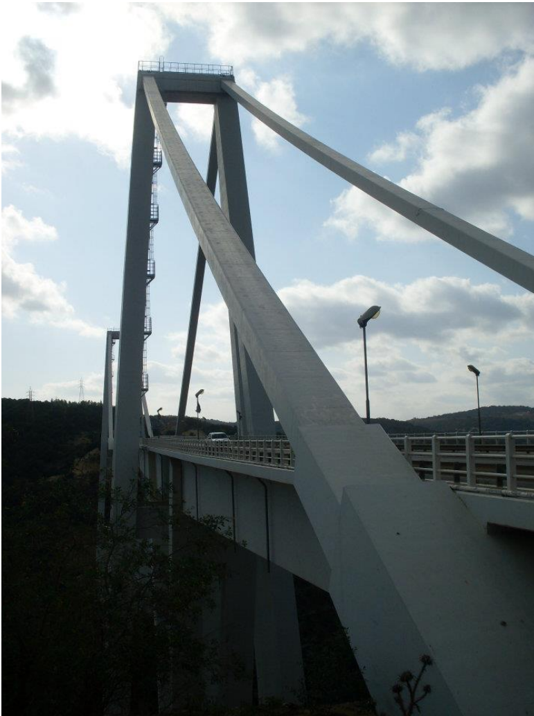
The Wadi al-Koof bridge. © Walid Tumi (ShababLibya 2011ah).
