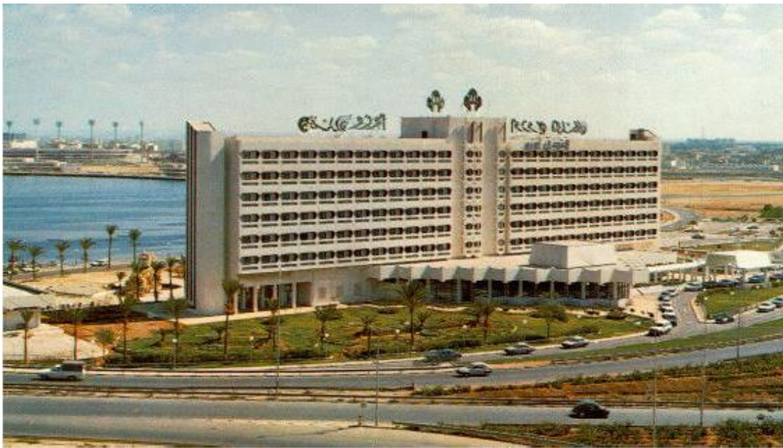
The Ozo Hotel in Benghazi (Libya Watanona 2019g).
