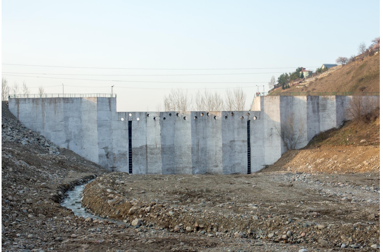
Image 4.2: Anti-mudflow dam on the Kargalinka River after the sel . Image taken by author.
