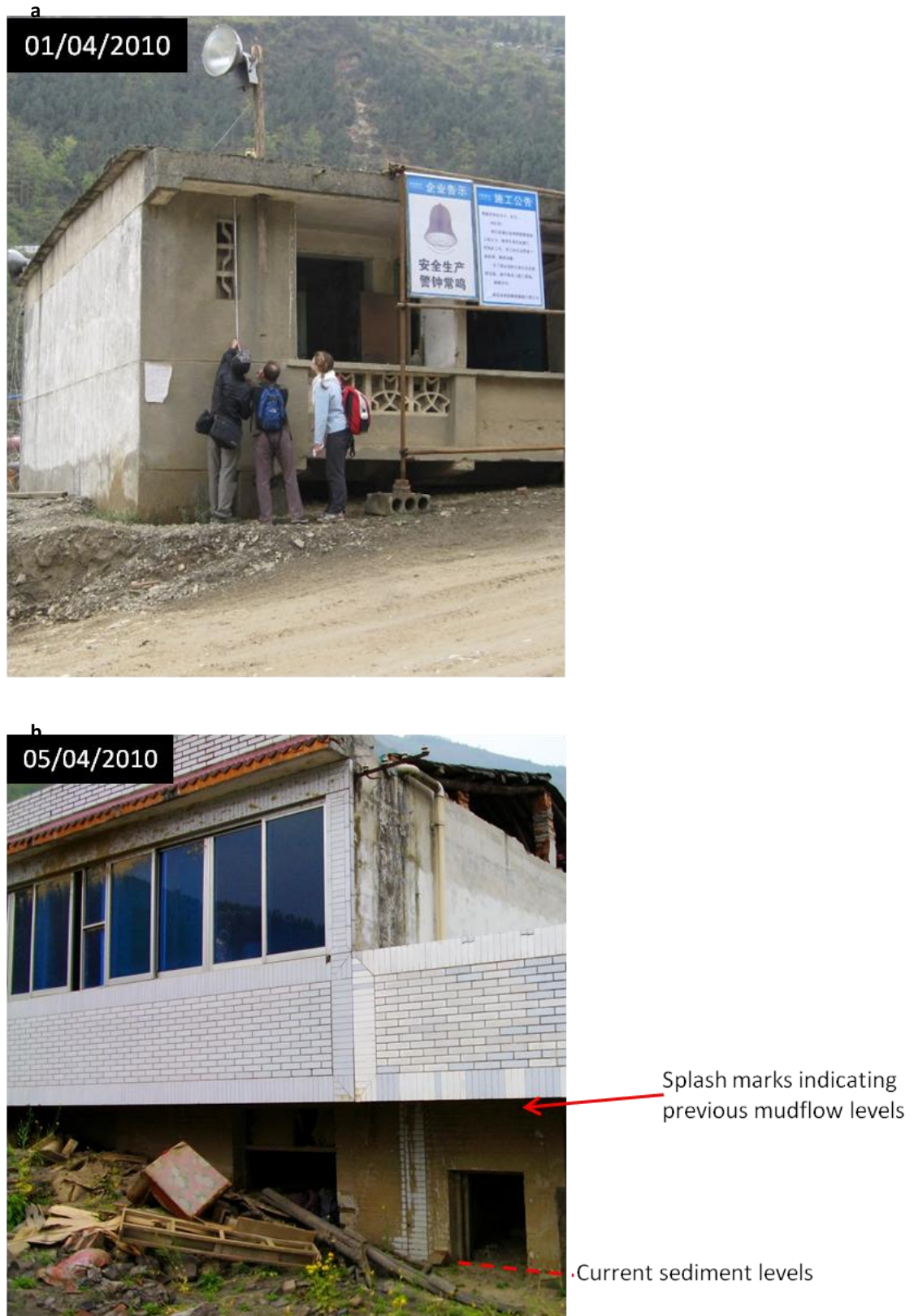
Figure 5.4: Photographs of fieldwork in Sichuan – a : measuring the floor height of benchmark buildings in Beichuan; b – assessing sediment depth (current and previous) in Huangjiaba.
