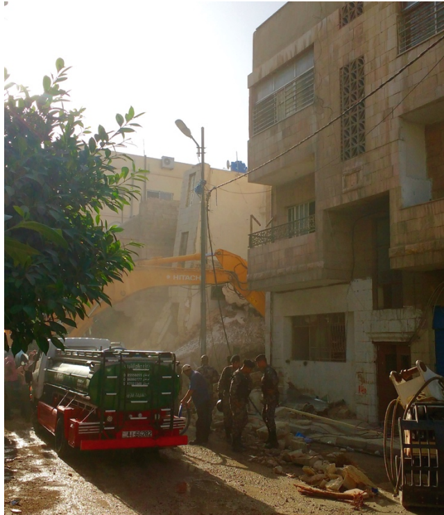
Fig.12 Building Collapse, al-Ghawariyah
