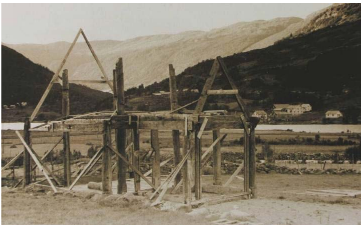
Fig. 42 Vang and Oye Stave Church. The top image is Vang Church in 1841. When parts were crated and sent to Poland for reconstruction, the entire roof structure is missing (drawing by Franz Wilhelm Schiertz). The bottom photo is Øye Stave Church during reconstruction. These are all that remained of the original structure. Both images used with permission from Riksantikvaren, Directorate for Cultural Heritage.
