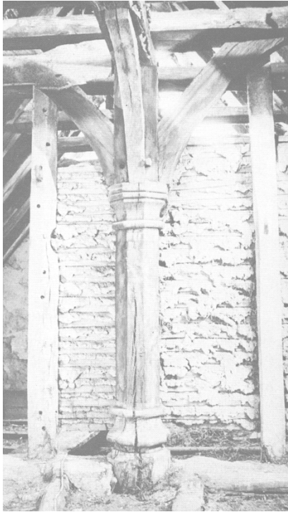
Medieval Crown Post (Netherdale, St Nicholas at Wade, Kent). Source: Harris 2012: Fig 11.
