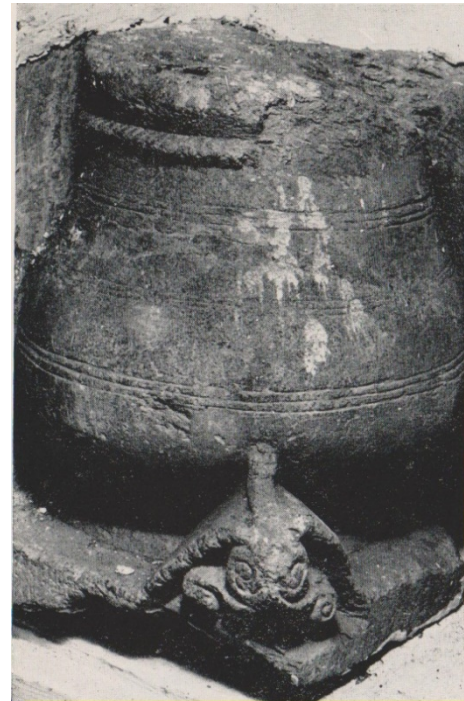
Fig. 40 Bulbous base from Haltdalen Stave Church. The image on the left is from Haltdalen Stave Church. The right hand image is a bell shaped base from Nidaros Cathedral. It is firmly dated to c. 1090-1120 (Photo source of Nidaros architectural remant from Blindheim 1966: Plate 11).
