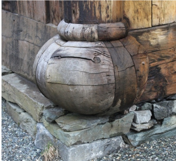
Fig. 40 Bulbous base from Haltdalen Stave Church. The image on the left is from Haltdalen Stave Church. The right hand image is a bell shaped base from Nidaros Cathedral. It is firmly dated to c. 1090-1120 (Photo source of Nidaros architectural remant from Blindheim 1966: Plate 11).
