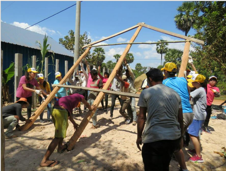
Figure 11 Everyone having their hands on the structure of the house at the moment of lifting it up
