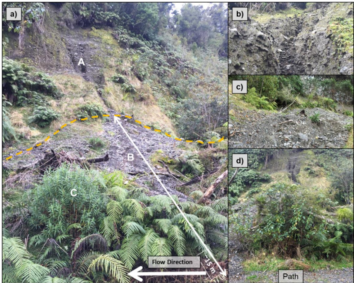
Figure 3.12. Photographs of Landslide 8. 3.12a. Landslide/Location 8 A: Landslide scar with two active gullies cutting into the bedrock. B: Conical Deposit. C: Woody debris and fallen trees litter the deposit surface. 3.12b. Displays the post-landslide erosion taking place within the landslide scar (A). 3.12c. A range of fresh woody debris and boulders make up the deposit. 3.12d. The landslide deposit is abruptly cut off by the access path.
