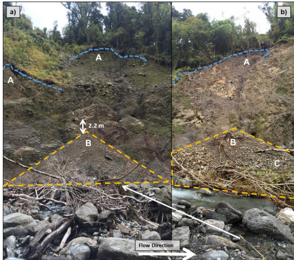
Figure 3.13. Annotated photographs of Landslide 9 and Landslide 10. The labels on both landslides represent the same characteristics. A: Steep, landslide scar and crowns (blue dotted line) exposing bedrock. Vegetation can be seen upslope of both scars. B: Conical deposits formed at the base of the hillslope consisting primarily of fine-grained material with some woody debris. C: Soil has been retained in the roots of the fallen trees in the deposit of Landslide 10 indicative of recent erosion. 3.13a. Landslide 9. 3.13b. Landslide 10.
