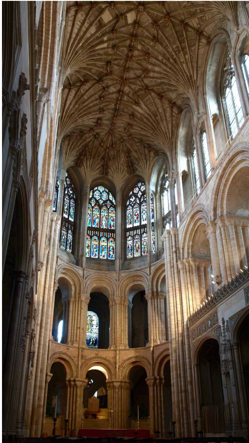
Figure 3.22: View of Norwich Cathedral's clerestory showing the stylistic disjuncture between the lower Romanesque arches supplanted by later Gothic arches above—a tangible result of the storm of 1362 and the repairs required in its aftermath. Photograph by the author.
