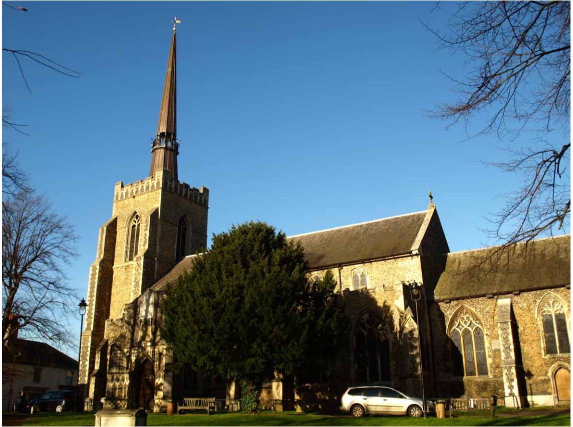
Figure 3.24: The church of St Peter and St Mary, Stowmarket, Suffolk. While the storm of 1362 is not specifically recorded affecting the building, the fact that the tower is constructed around a timber framework dating to 1362/3 and later documentary evidence describes it as the new tower, strongly suggests the St Maur's Day storm damaged the tower which was repaired in the aftermath. The current spire is a replacement for one blown down by the great storm of 1703 Photograph by the author.
