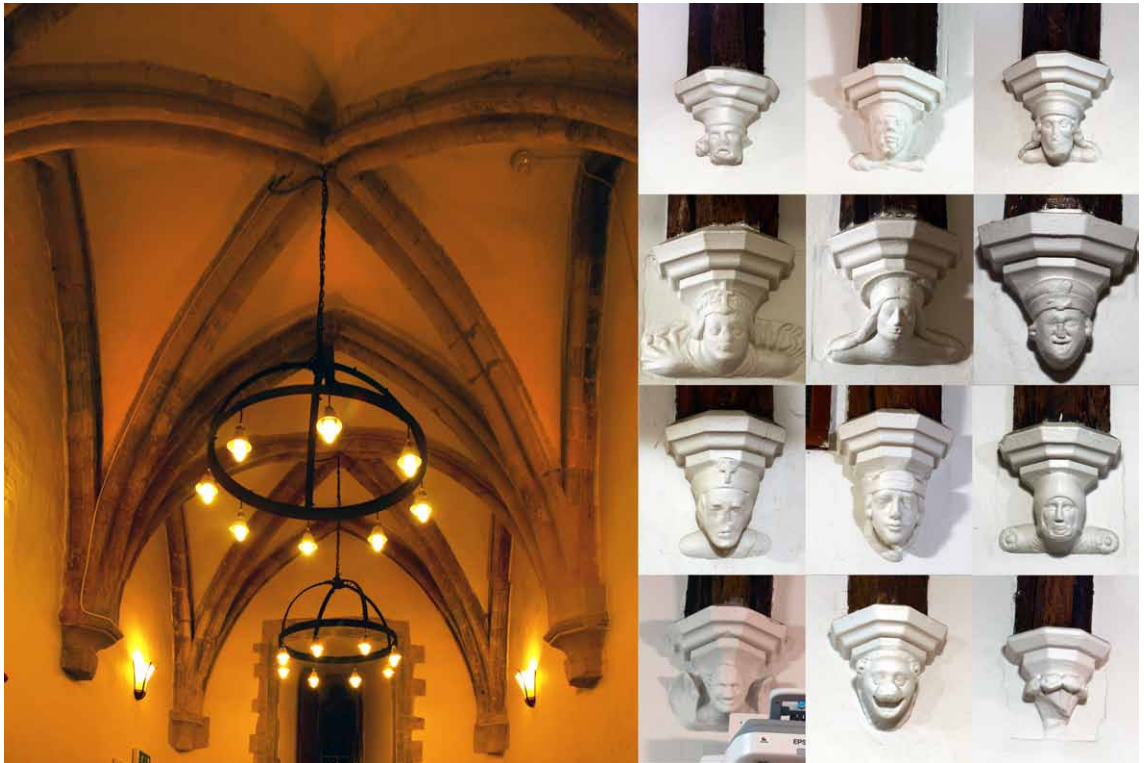
Figure 4.7: Left: Rib vaults in one of the ground floor chambers. These date stylistically to the 13 th or early 14 th century and therefore predate the storm of 1362. Therefore, they must have been re-purposed from an earlier structure. Right: Decorated corbels now located inside chambers on the second floor of the gatehouse of St Albans Abbey. Although these were similarly thought to pre-date the storm, close parallels with other late 14 th century sculpture suggests they are more likely to relate to the reconstruction phase in the storm's aftermath. Photographs by the author.
