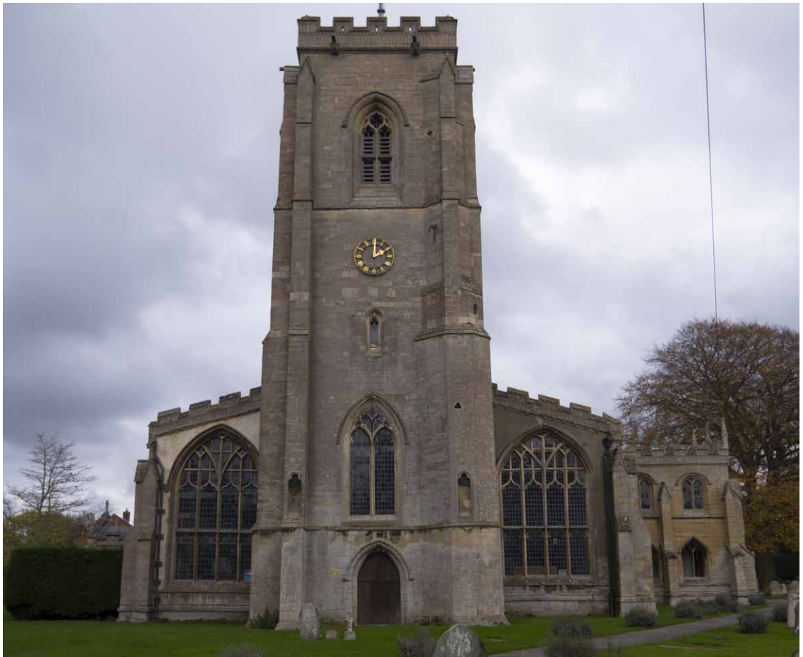
Figure 3.13: The west front of the parish church of Walpole St Peter, Norfolk. Note the clear distinctions between architectural phases with the original tower, constructed in c. 1300 (the only surviving part of the original church with the rest thought to have been swept away in a marine inundation), the later nave dating to the 1360s and the later south porch ( c. 1425) on the right-hand side. Photograph by the author.
