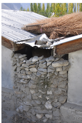
Coarse stone masonry wall constructed between shelters to protect items in Aliabad.
