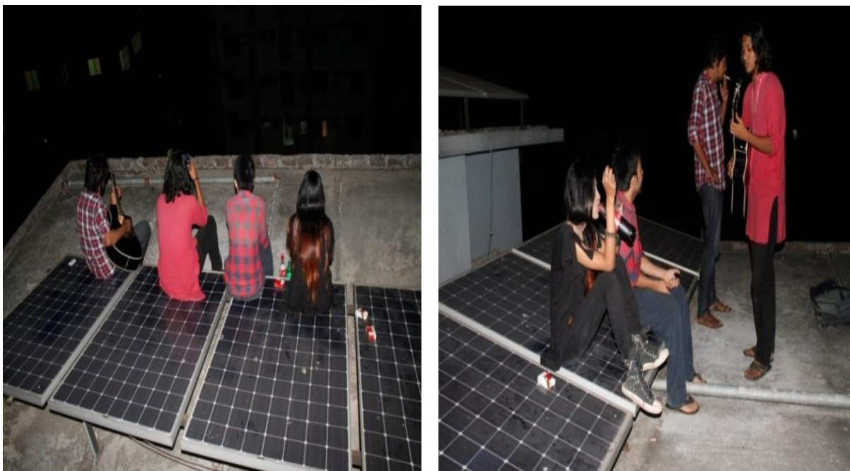
Figure 8:9 Out of service solar panels Source: Author
