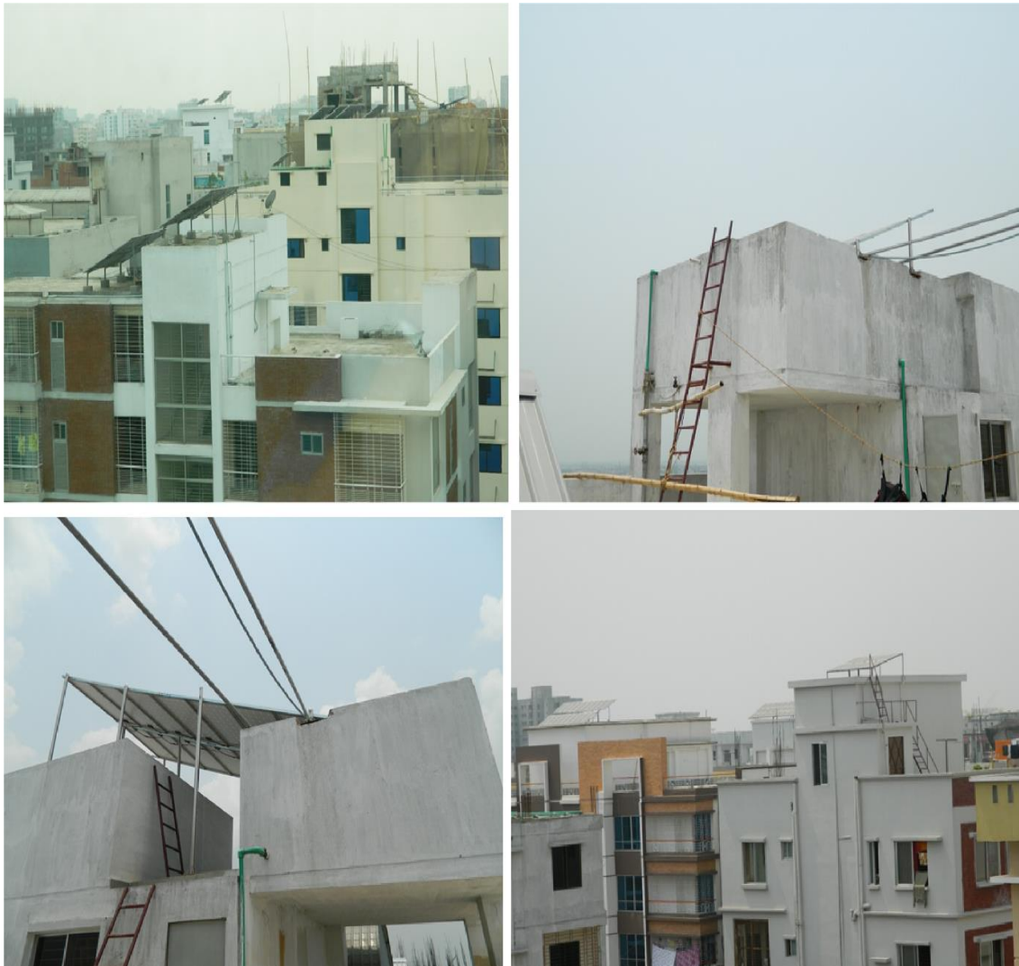
Figure 8:8 Solar panels on rooftops
