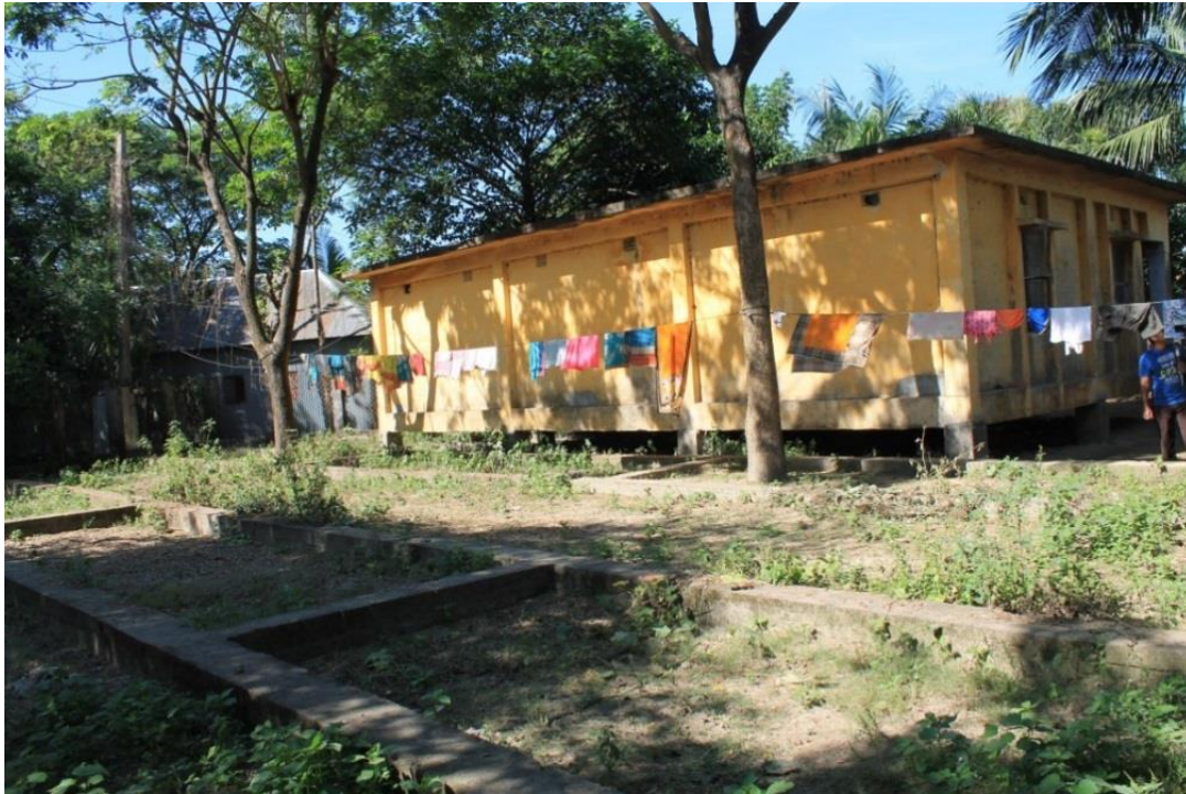
Figure 3:5 Former solar panel station in Narshingdi. Source: Author
