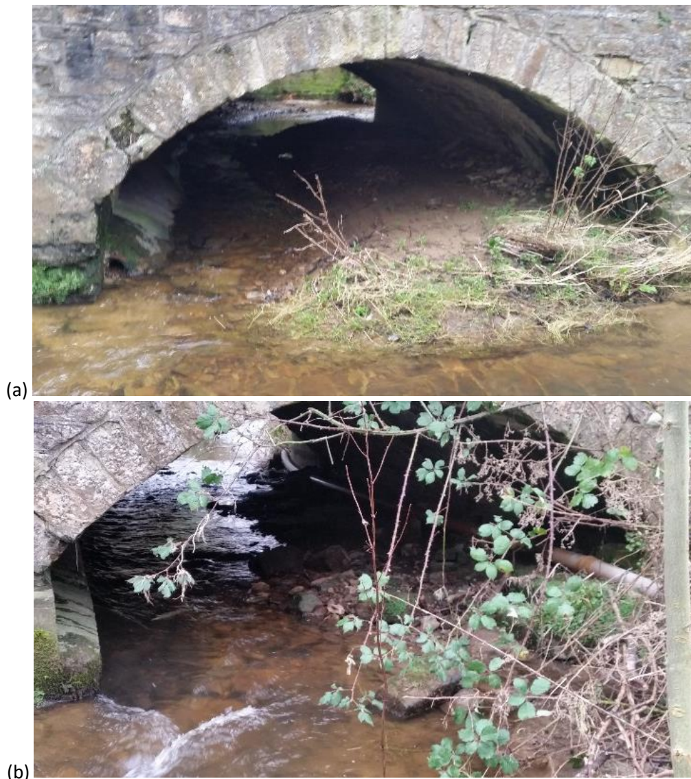
Figure 9.2 Image showing the two bridge spans (a) eastern span; (b) western span (author, 31 January 2016).
