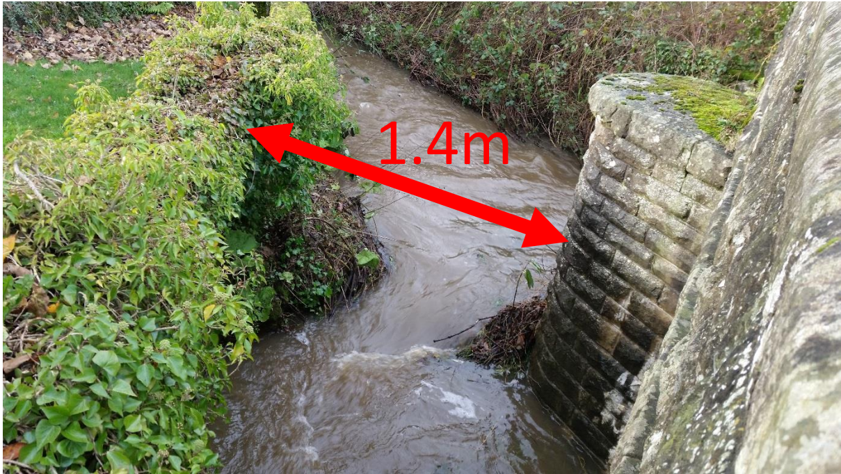
Figure 9.1 Image showing the confined entry into the eastern span because of the bridge widening (author, 15 November 2016).
