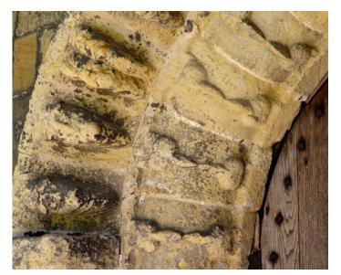
Fig. C.33. Salton, St John of Beverley (North Yorkshire): eroded beakheads on the south nave doorway.
