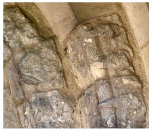
Figs. C.37 & 38. Sherburn, St Hilda (North Yorkshire): badly damaged beakheads on the reset south nave doorway.
