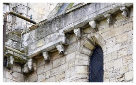
Fig. F.22. Selby Abbey: eroded corbels on the exterior of the north nave and north transept.
