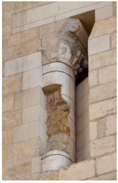
Fig. B.8. York Minster: column embedded in east wall of the south transept (interior).
