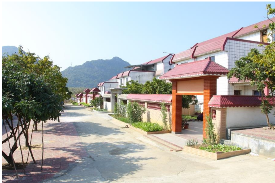
Figure 2.11: Typical Housing of Baikou New Village
