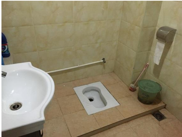
Figure 7.22 Weishengjian with a squat toilet
