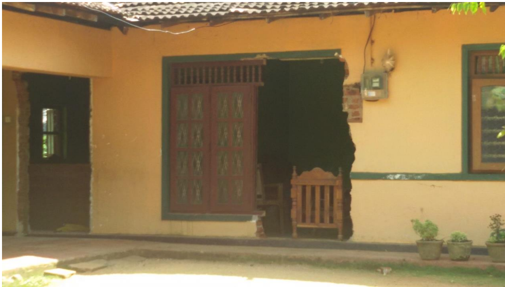
Figure 11 The Gaps in Front of Premalatā's Gedara
