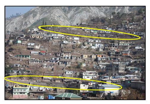
Figure 5.18 Massive building and road construction (yellow circles) on steep slopes in Muzaffarabad city. All the construction has been done after doing earth cutting.
