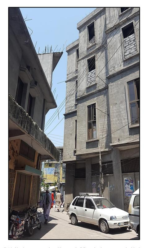
Figure 7.14: Newly constructed multi-storey buildings in the congested old city area of Muzaffarabad. Notice narrow street and addition of new storeys on an old dilapidated building on the left.
