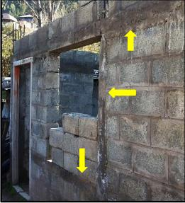
Figure 7.1 (left) An under-construction pukka house in rural Bagh with no plinth and lintel level beams in walls (yellow arrows) in contravention to the ERRA specifications; (right) a seismically compliant under-construction *pukka* house in rural Muzaffarabad with proper pillars and beams. (Source: Author fieldwork)
