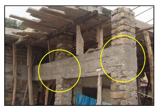
Figure 7.2 An under-construction house in Muzaffarabad city; notice brick columns and concrete beam in utter violation of the engineering principles (yellow circles).
