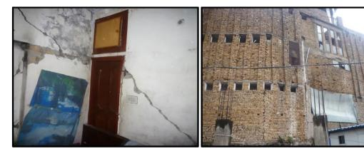
Figure 7.7 A damaged house in Bagh city which has been partially repaired and still inhabited by the owner and his family (left). A pre-earthquake multi storey commercial building in Bagh city, non-frame structure and cracked walls pose serious threat (right).
