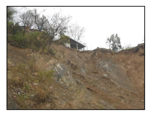
Figure 7.17 A house facing immediate collapse due to landslide in Lohar Gali area of Muzaffarabad District. (Source: Author fieldwork)
