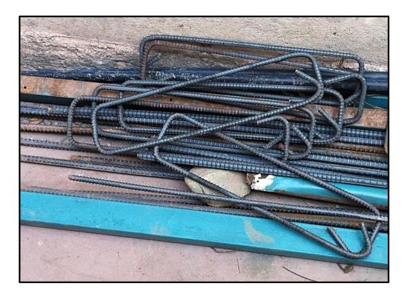
Figure 7.3 Properly formed steel rings for RCC frame structure, a rarity before the earthquake. (Source: Author fieldwork)
