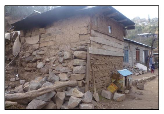
Figure 7.8 A poor quality structure (foreground) added with a reconstructed house (background) in Bagh city; notice different types of materials and irregular stones used in the added structure.
