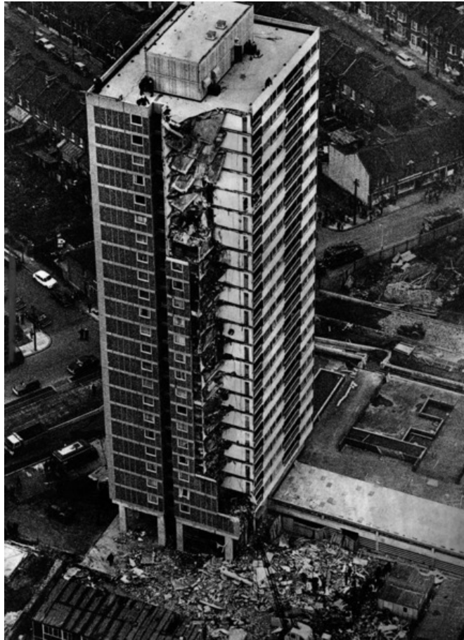
Figure 11 - Photograph of Ronan Point, 1968
