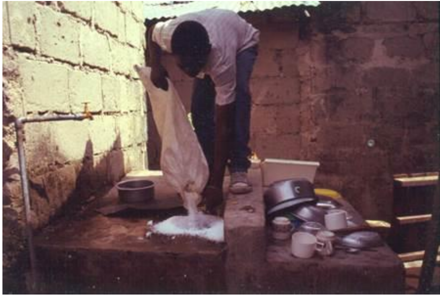
Figure 4.2: Treatment of latrines with expanded polystyrene beads (courtesy of J. Ensink)
