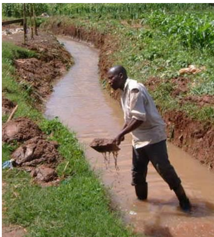
Figure 5.2: Environmental management through drain clearing to reduce breeding sites (photo courtesy of S. Lindsay)
