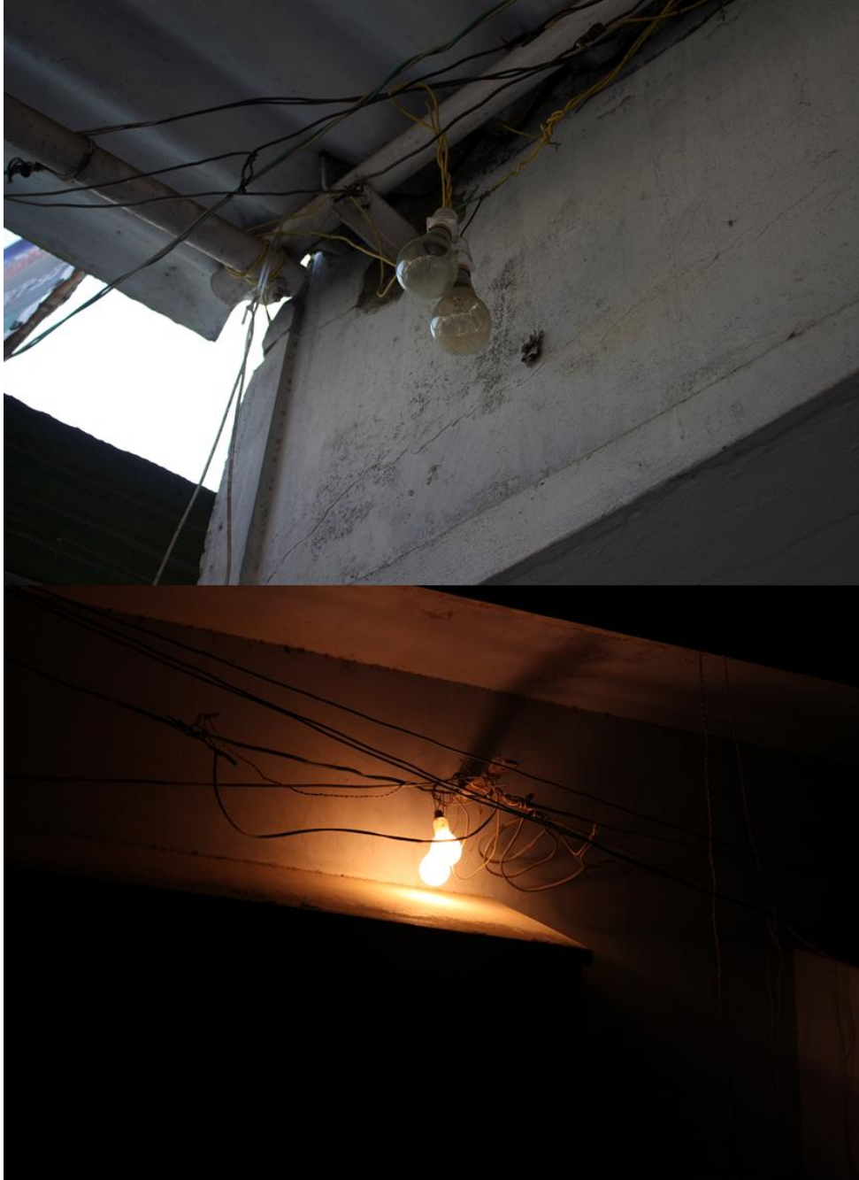
Figure 7-7: Bulbs used as 'choke points' by HPS.
